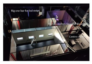
One bar needs to be rigged in the back of the installation for two Led strips
